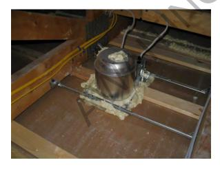
Air sealing is discovering all the nooks and crannies that allow air to leak in and out of the home and sealing them up! Gaps and open seams can form along the edges of doors and windows and even around the can lights in your sealing.
