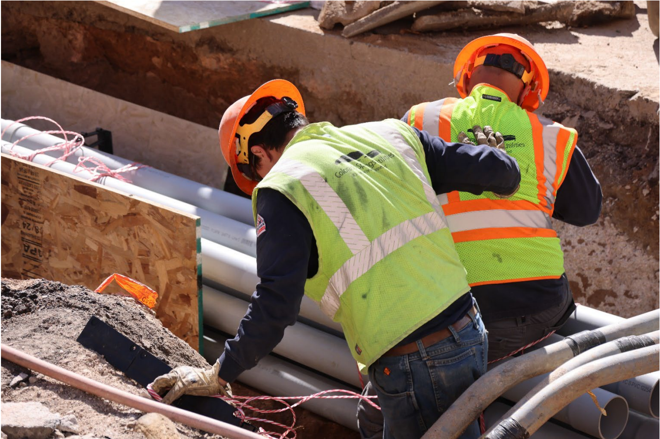
Photo 4 – Example of new underground conduit
