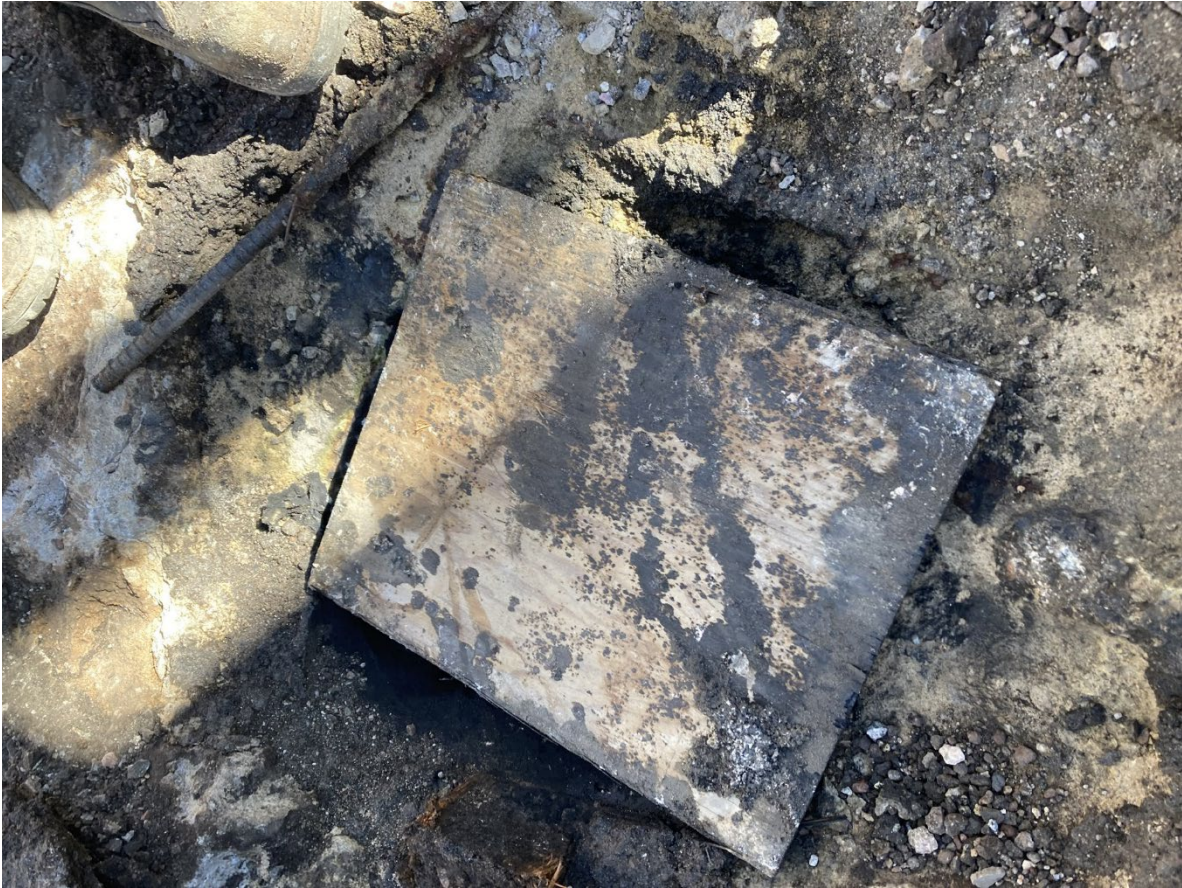
Photo 1 – Plywood patch
