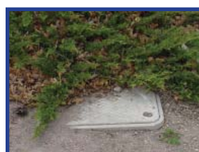
Inadequate clearance
