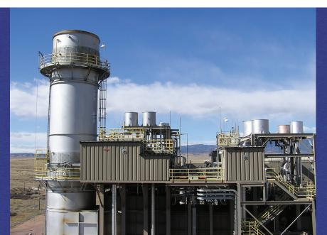
The Front Range Power Plant operates on a combined-cycle system producing up to 50 percent more electricity than a traditional plant.
