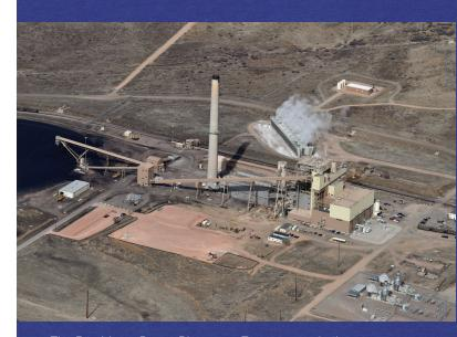
The Ray Nixon Power Plant near Fountain was built initially to burn coal, and gas-fired combustion turbines have been added.
