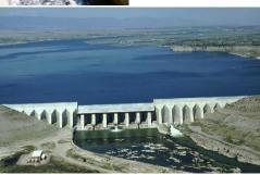
**Dam**: Used to create a reservoir which stores water.
