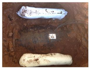
Cathodic protection installed on a 20' water pipe.
