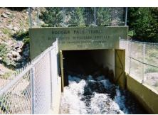
**Tunnel**: A belowground channel used to transport water from other areas. Our tunnels move water through the Rocky Mountains.
