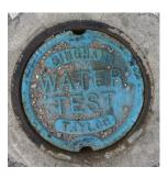
General: The Water CP Test Station offers the versatility of being buried in or near street pavement. Each 5.25-inch lid shall be painted "Blue" and shall have "Water Test" cast into the Heavy Duty H20 rated lid. The body shall be 15 inches in height and made of high impact plastic. A 5-terminal test board shall be attached to the lid. This test box will be used in conjunction with Cathodic Protection Test points and systems.
